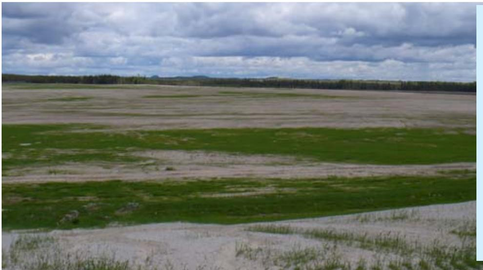
At the abandoned Kamkotia Mine in Ontario tailings that were originally discharged into an impoundment and freely onto the land and are now being rehabilitated using a dry cover. The large area of tailings in this picture is only one of tailings management areas. As this site was abandoned Ontario tax payers are covering the \$60-million cost of rehabilitating this site.
